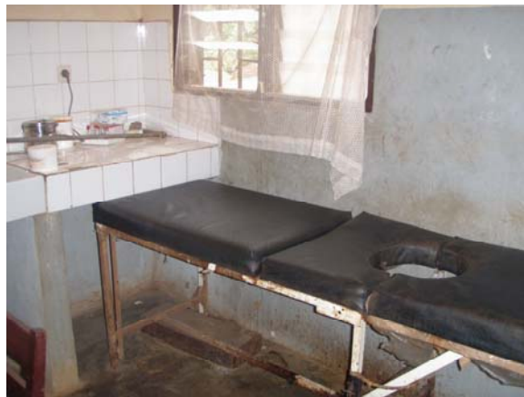
Photo 6 The delivery room in the health centre of Asung
