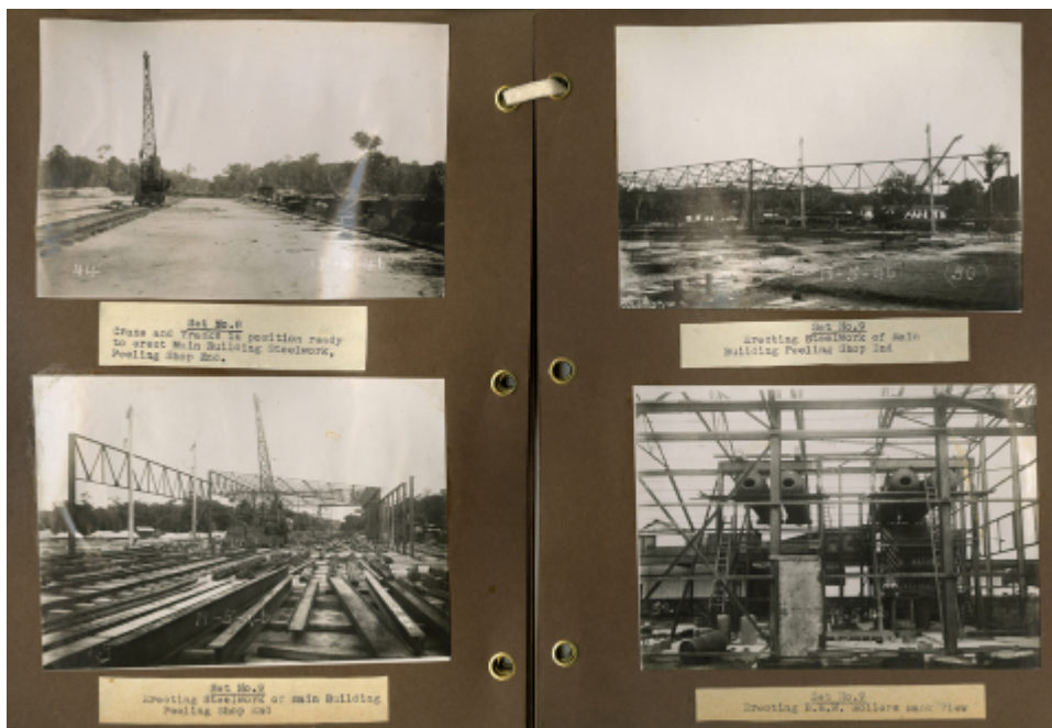
Figure 8: Construction of the Sapele Sawmill, Nigeria, 1946.
