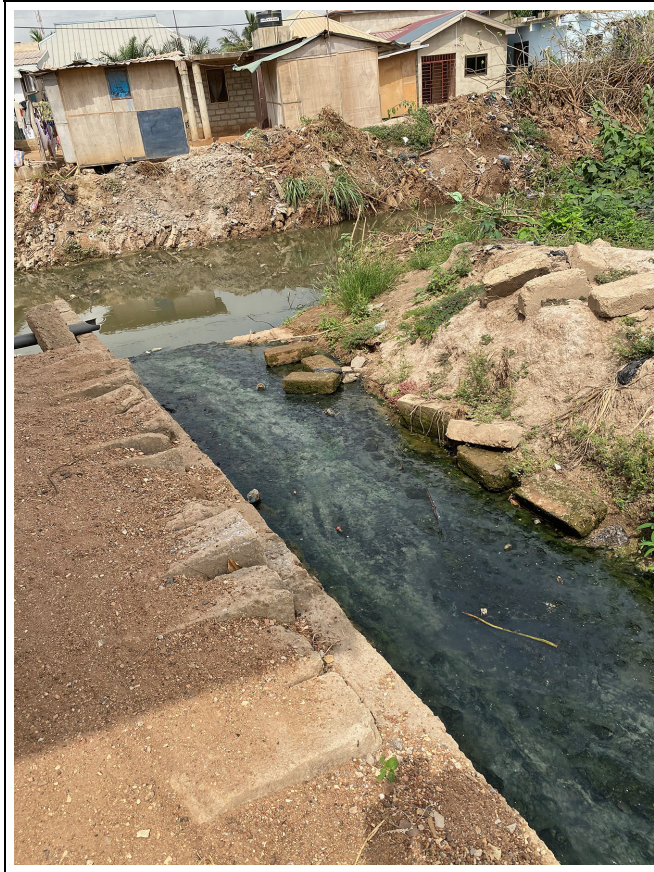
Figure 3. Drain constructed by group of residents, western end of Tuabodom, 2021.
