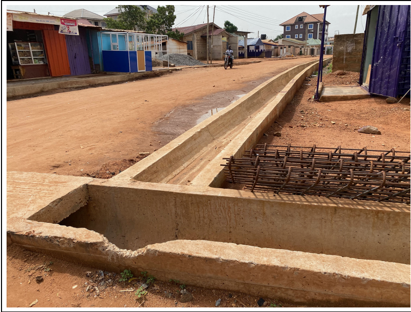
Figure 4. Newly constructed roadside drains in Tuabodom, 2022.
