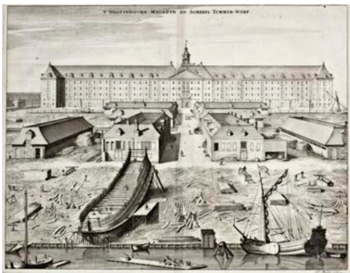
*Fig. 9. The shipyard of the VOC (Dutch East India Company) on Oostenburg in Amsterdam; on the background the large East Indian Sea Warehouse and slipways on the foreground (print J. Mulder, 1694, from Commelin 1694).*
