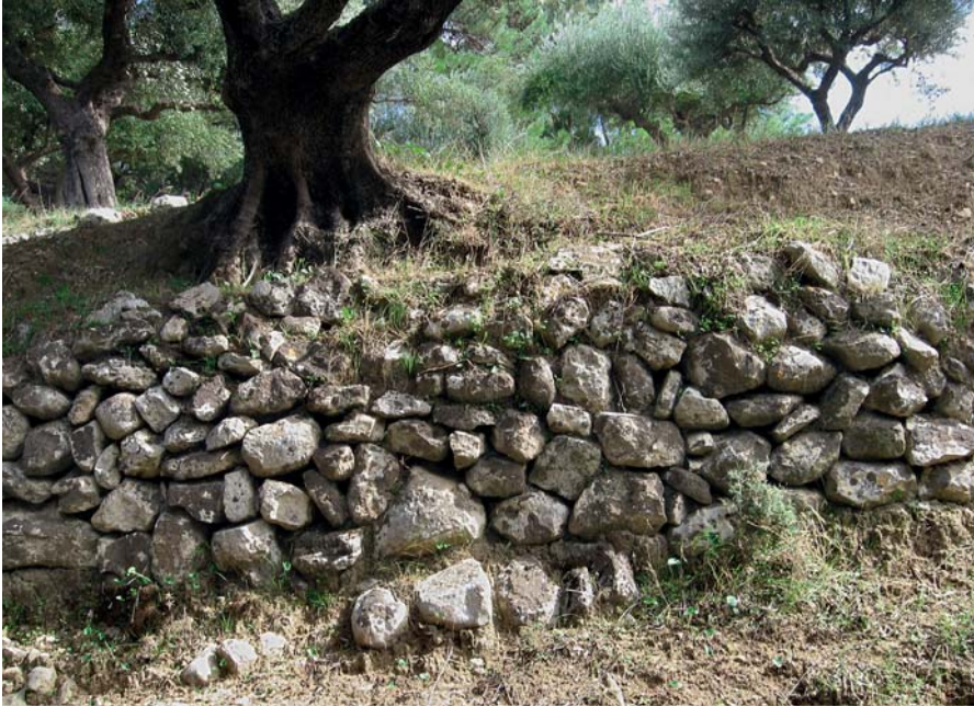
Figure 10. Terrace wall on the western slope of Kokkala hill that incorporates parts of older walls
