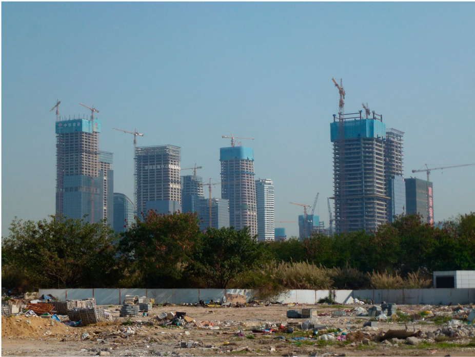
Figure 3. Qianhai under construction. Photo by author, 2018.
