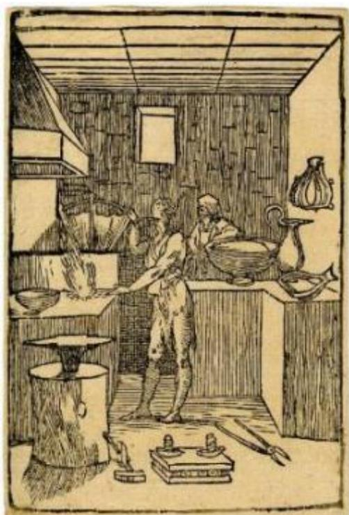
Fig. 1.11. Domenico Beccafumi, c.1540-1550. Woodcut illustration of a silversmith in his workshop. From a series of ten prints: *The various operations of alchemy*. Empty casting flasks are seen hanging on the right wall, on the work bench on the right and filled flasks are visible in a clamp on the foreground. (image British Museum)
