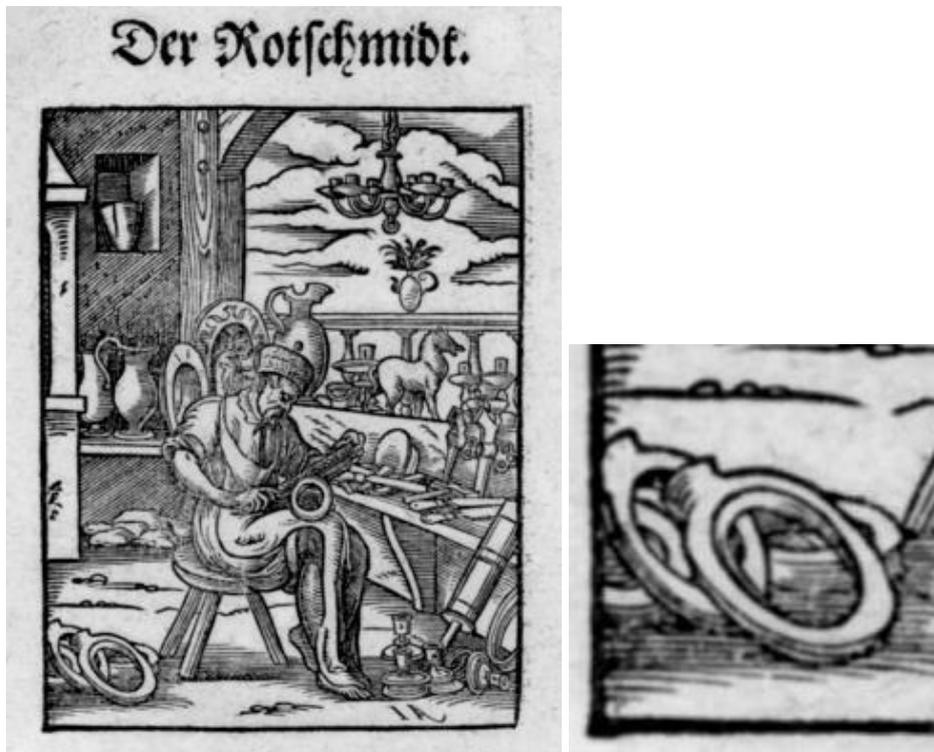
Fig. 1.16. Jost Amman, *Der Rotschmidt*, 1568. A woodcut illustration of a brass foundry. From Hans Sachs, *Panoplia omnium liberalium mechanicarum et sedentariarum artium genera continens*, Sigmund Feierabend, 1568. On the right a detail of the metal flasks used for sand mould casting.
