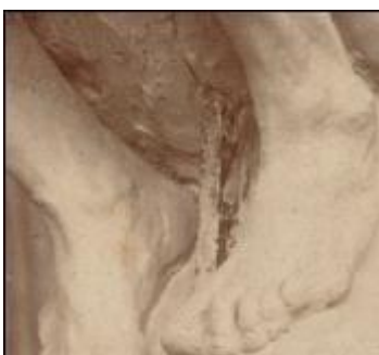
Fig. 3.7. detail of Ph 01020 showing the protruding part of the armature.
