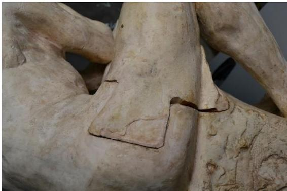
Fig. 4.8. Detail of foundry plaster S.2840, showing the dovetailed joint.
