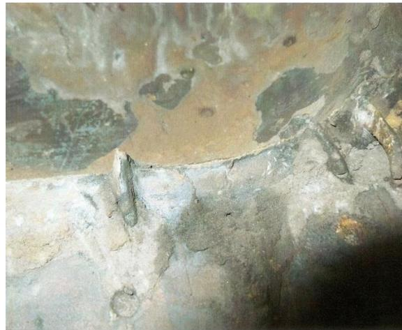
Fig. 4.40. Reinforcing ribs on the interior surface of the Washington *Thinker* (image National Gallery of Art Washington)
