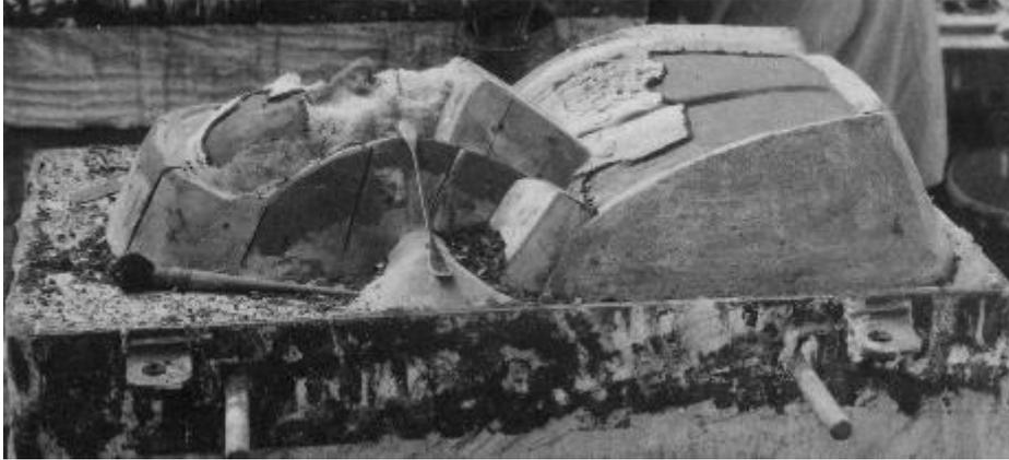
Fig. 4.38. The cutting back of the core of a bust in progress. (image taken in unknown foundry, probably French first half twentieth century, image private collection)
