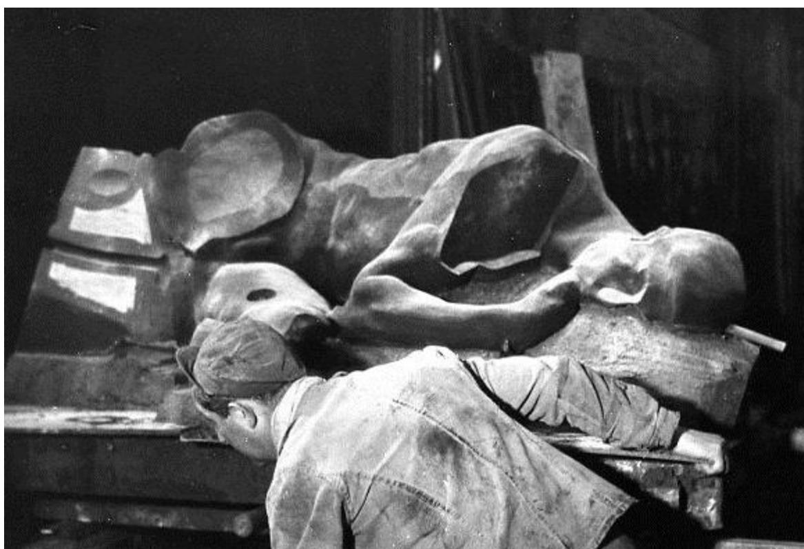
Fig. 4.41. Robert Doisneau, silver gelatine print, Paris, 1950. The core of the monumental *Thinker* during moulding in the Rudier foundry. Note the lantern protruding from the top of the skull. (image Doisneau estate)
