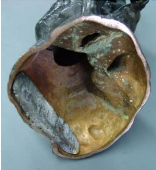
Fig. 4.92. Interior view of the base of the reduced size *Thinker* (private collection) with the counterweight. (image Rupert Harris)
