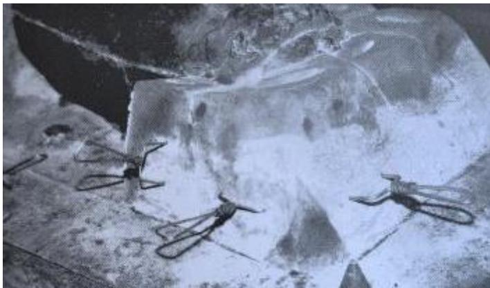
Fig. 4.30. Manipulation of false-cores with the aid of core-pins. (from Rama 1988, 143)
