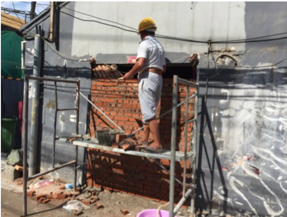
Figure 4.3 ‘Bricking up the hole’ (Photo by author, 2017, Beijing)
