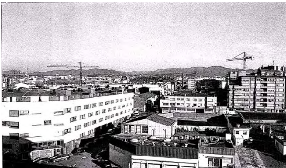
Figure 4: Construction cranes on Terrassa skyline
