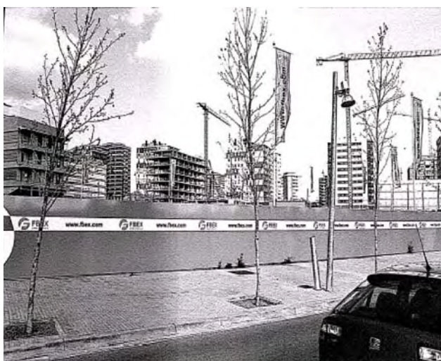
Figure 7: Can Palet construction site
