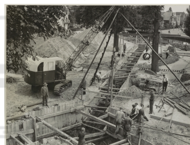
(c) Construction Site.
