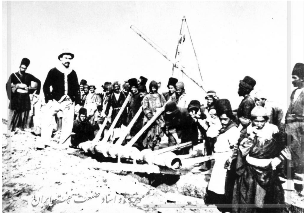
Figure 7.9: Photograph showing workers fitting an underground oil pipe 536
